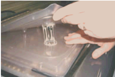
Take off old sprinklers
